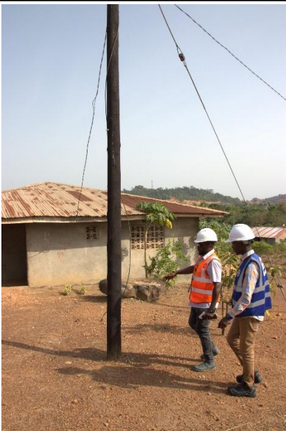
Joint inspection of light pole
