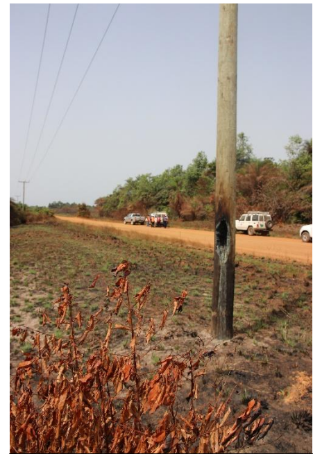
Wooden pole damaged by bush fire
